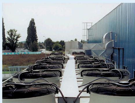
The condenser units are positioned on the roof, directly on top of the central refrigeration system. In the background: central ventilation unit.
