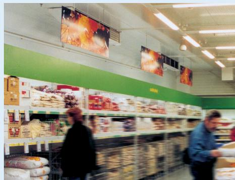
Single discharge ceiling mounted "low noise" model GDF air cooler with reduced rotation speed, for low-noise cooling.
