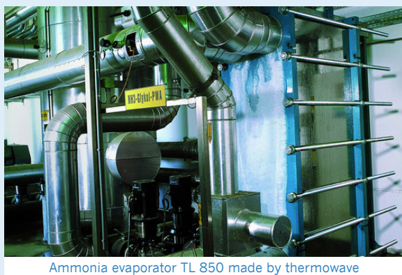
Ammonia evaporator TL 850 made by thermowave
